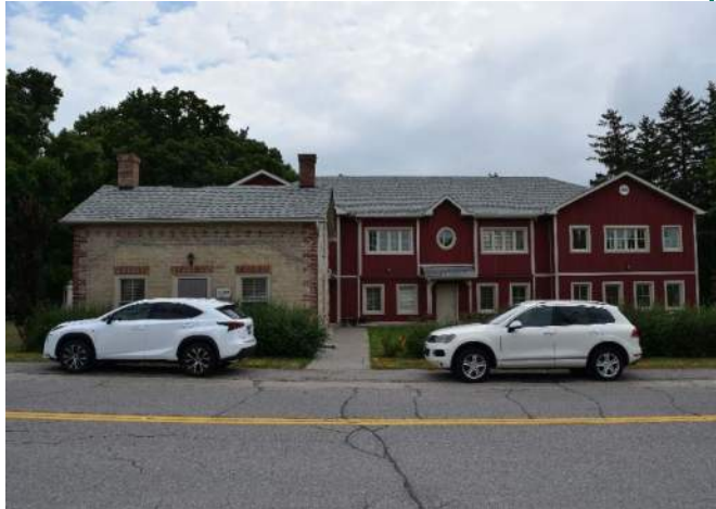
View facing east
