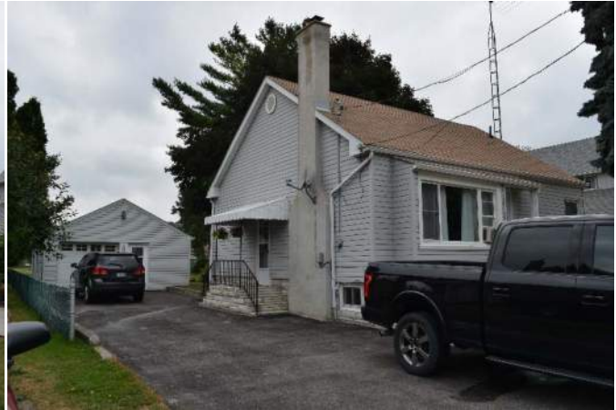
View facing northwest
