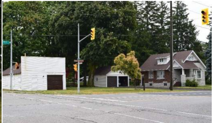
Garage, secondary structure and house at 3026 Elgin Mills Road
