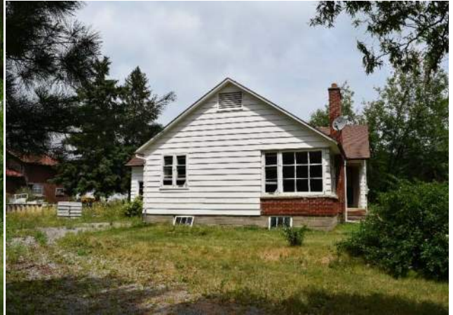
View facing north. The red-painted secondary structure can be seen at far left.
