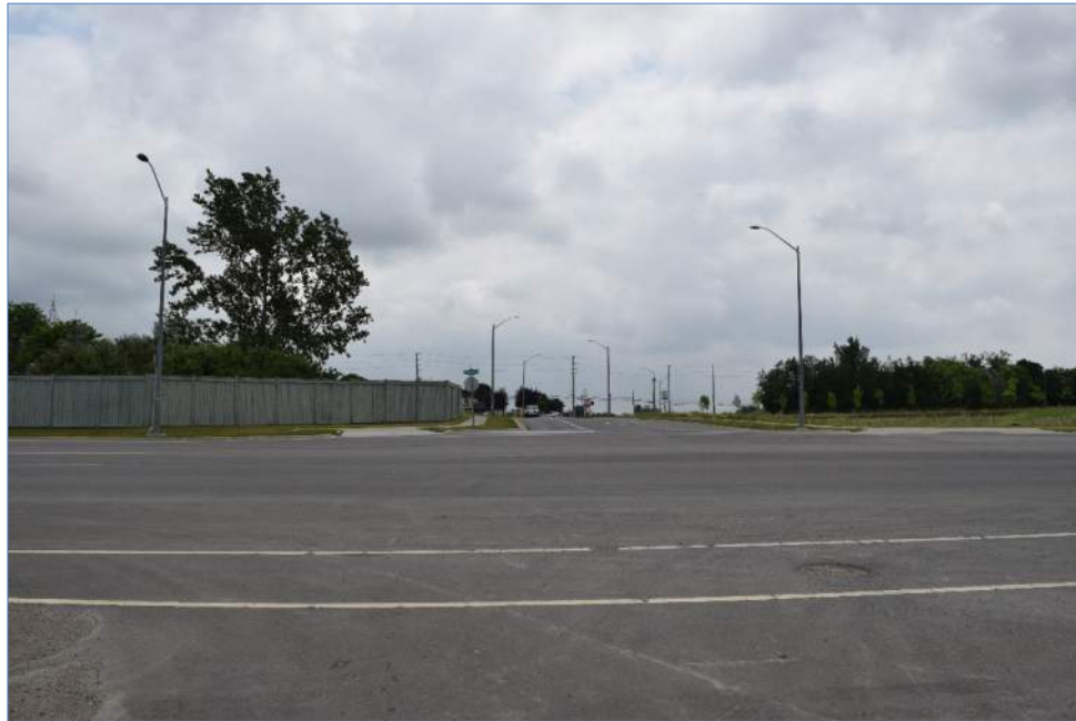
Figure 9: View facing east of the north connection of Woodbine Bypass and Victoria Square Boulevard.
