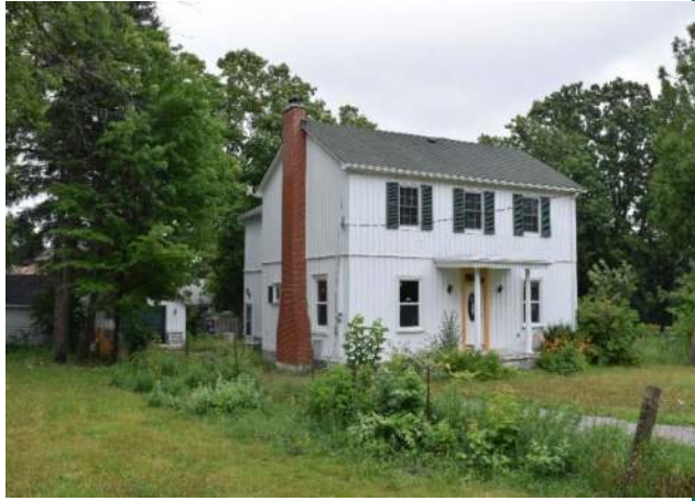
View facing southeast. The secondary structure can be seen at left.
