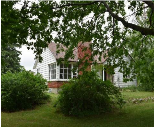
View facing northwest
