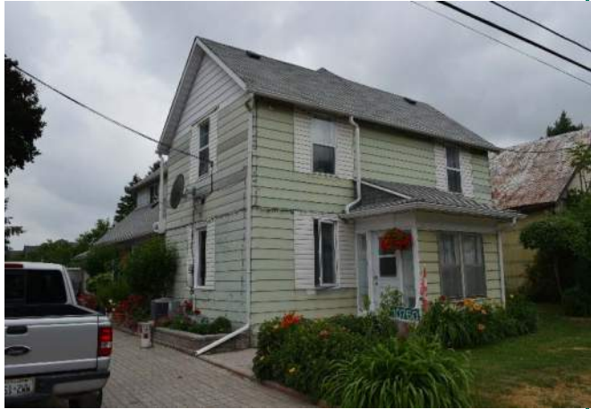
View facing northwest
