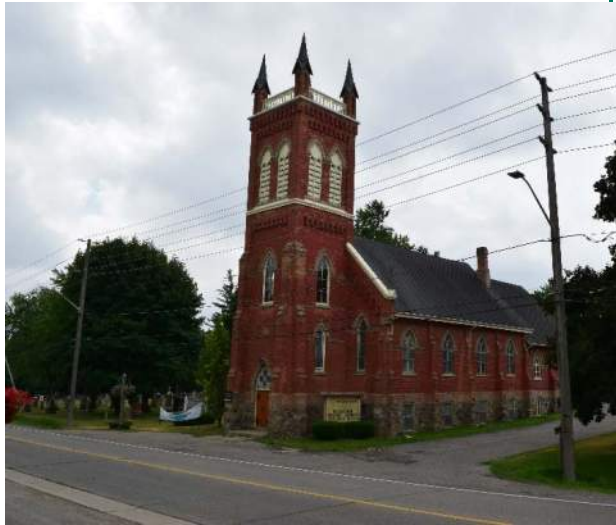
View of the United Church facing southwest
