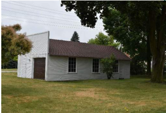
View of garage facing northwest
