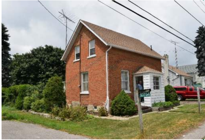
Above: View facing northwest
