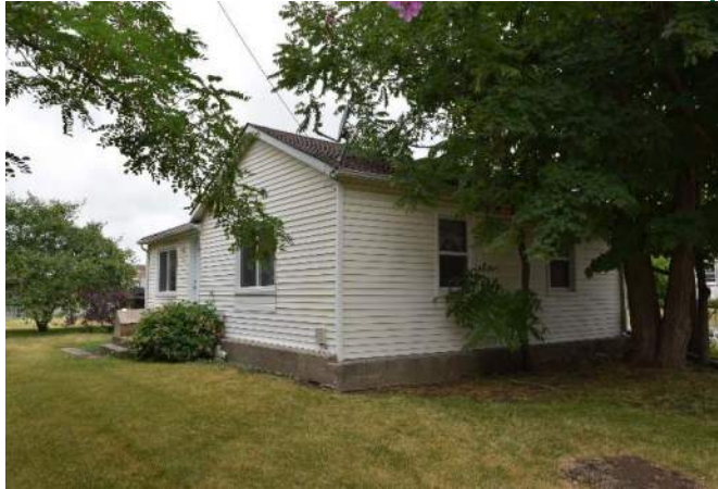
View facing northwest
