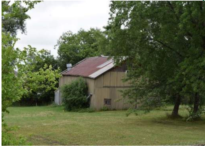
View facing east
