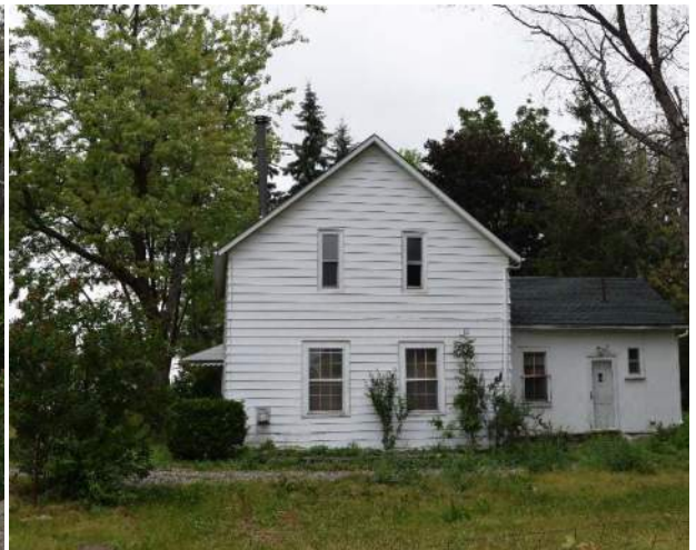
View facing north
