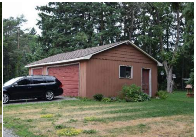
View of the shed, facing west
