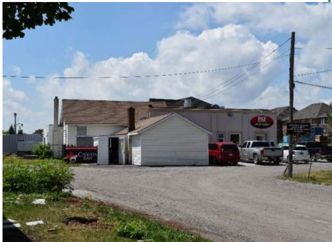
View of shop southwest of Herman Boynton House
