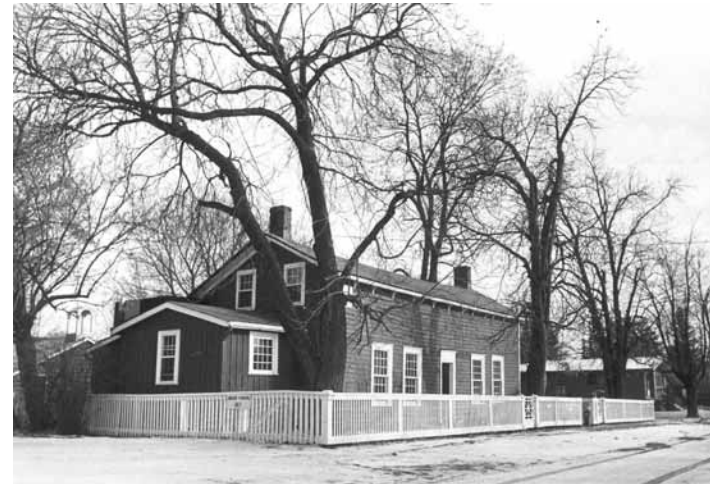
Traditional picket fencing reintroduced, 14 Colborne Street, Weaver #88.
