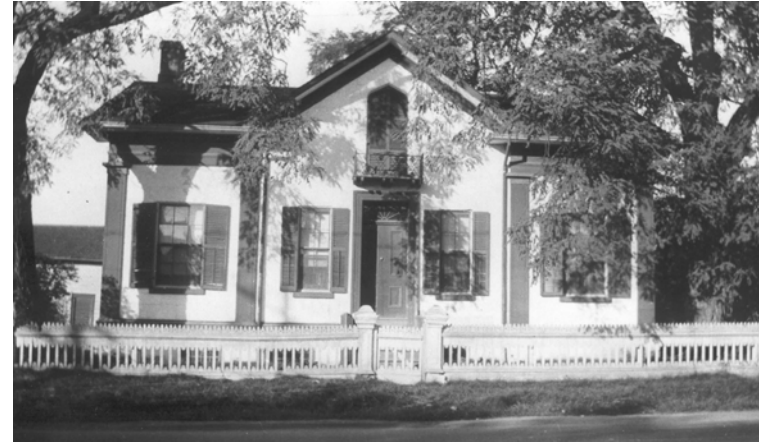
Fencing at the Edey House, 7690 Yonge Street (since moved to 44 Leahill Drive) Weaver # 399.
