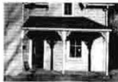
Simple Vernacular veranda
