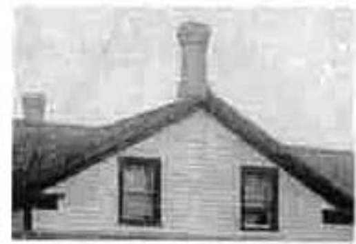
Simple Classic Revival cornice and returns
