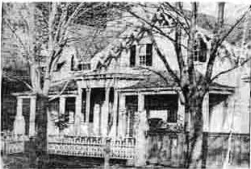
The Unionville Vernacular Salem Eckardt House, 197 Main Street
