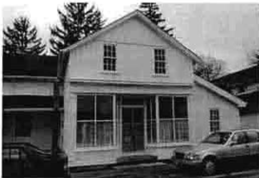
Vernacular gable-end commercial building, 154 Main Street Unionville
