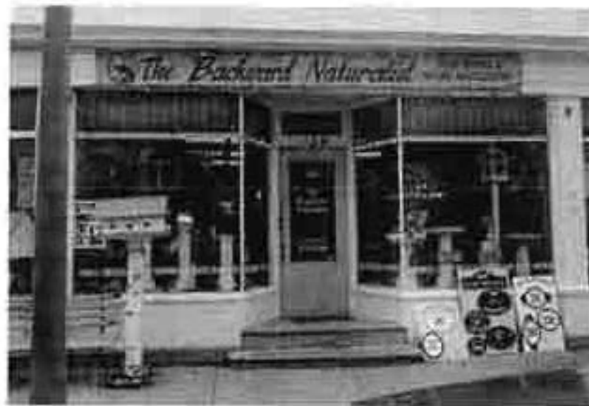
Typical Unionville storefront with recessed entrance, 156 Main Street
