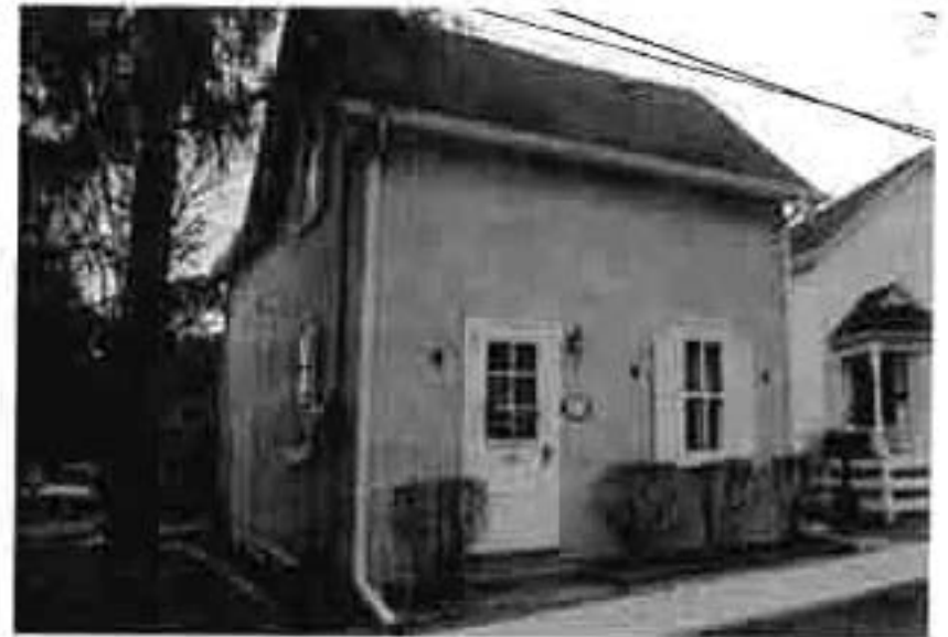
Vernacular workers cottage, 27 Victoria Avenue
