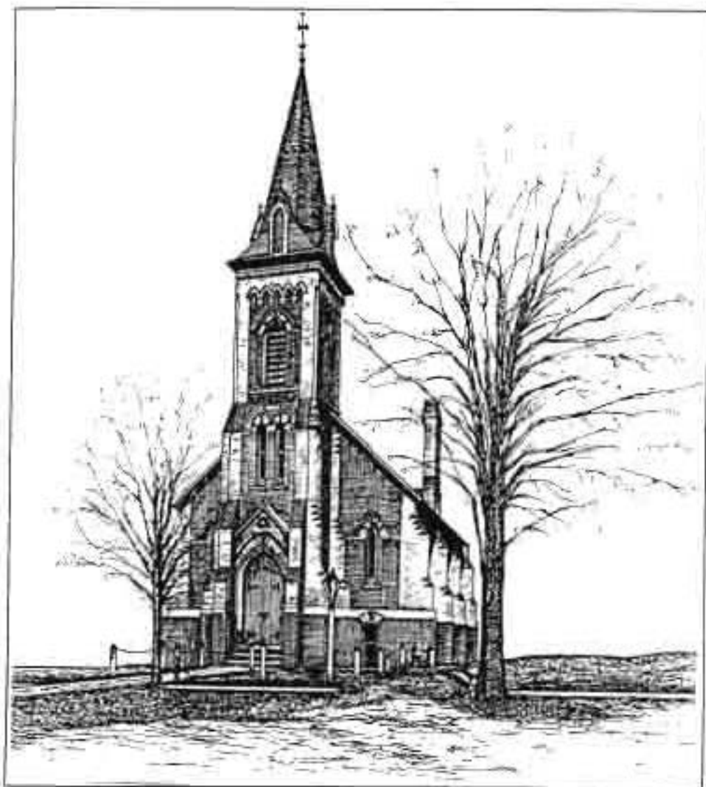
Central United Church, 131 Main Street Unionville
