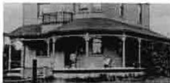
Late Victorian wrap around veranda
