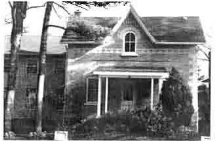
Gothic Revival cottage with multi-chromatic brick, 33 Union Street
