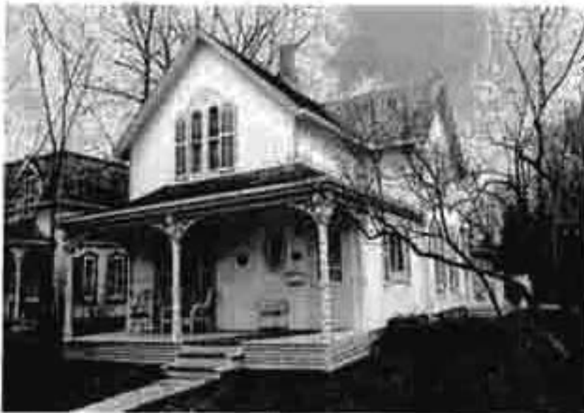
Italianate cross-gable house, 121 Main Street
