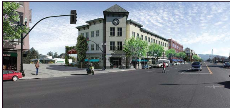
Photograph of existing development site(top).
