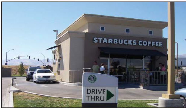
Big-box retailer (above); Drive thru (below).
