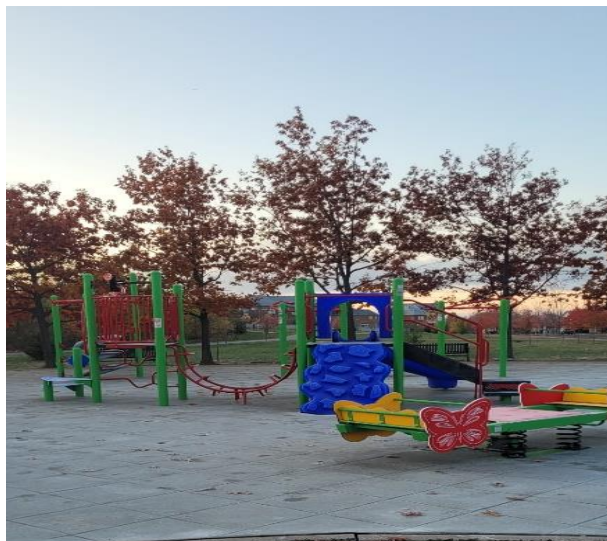
Playground and Rubberized Surfacing replacement
