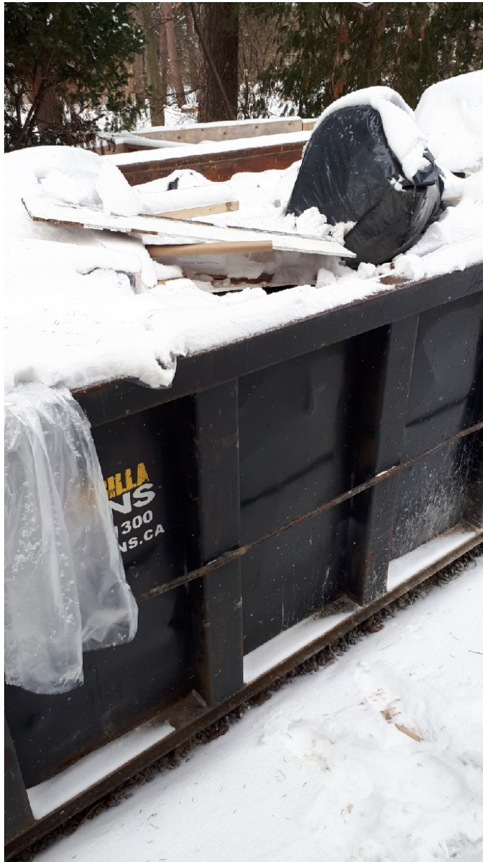
Bin With Previous Clapboard Siding – January 22, 2019
