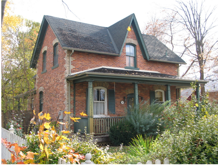
Front View (west)
