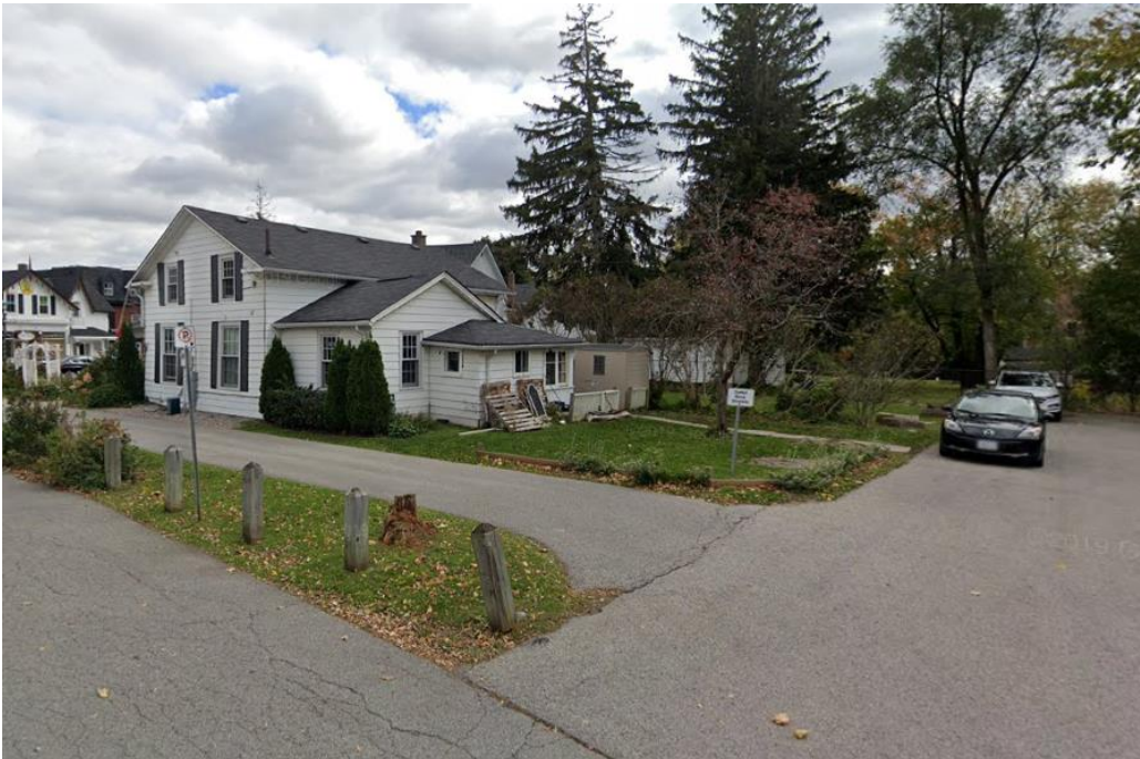
North and west (rear) elevations of the commercial building on the Subject Property (Source: Google)
