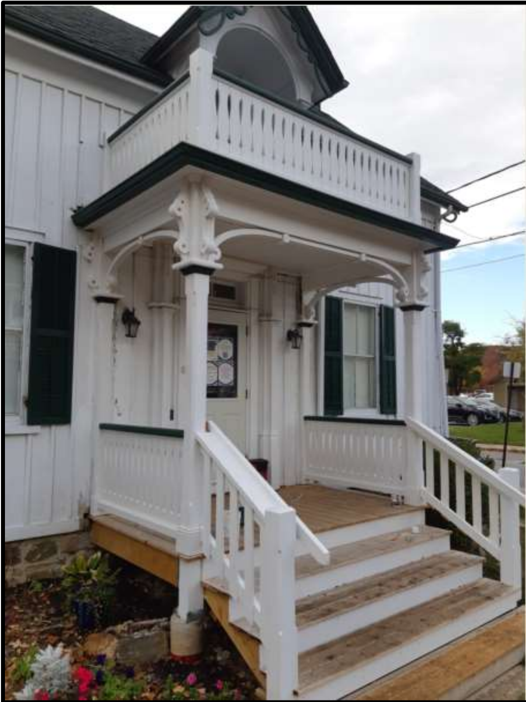
Figure 3- Photograph of newly constructed front porch and steps
