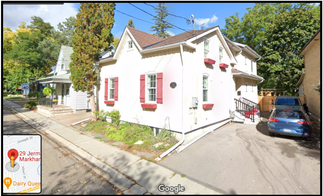
FIGURE 2-PHOTOGRAPH OF THE EXISTING HERITAGE DWELLING
