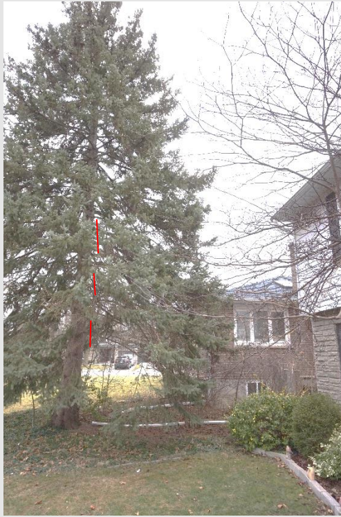
Image looking southward from the front yard shows the dwelling to be demolished (far right), shows the 42.5cm dbh white spruce (tree #2) to be protected with professional crown pruning (cuts in red) to provide adequate dwelling construction clearance, followed by tree protection fence installation (foreground), and root pruning works.
