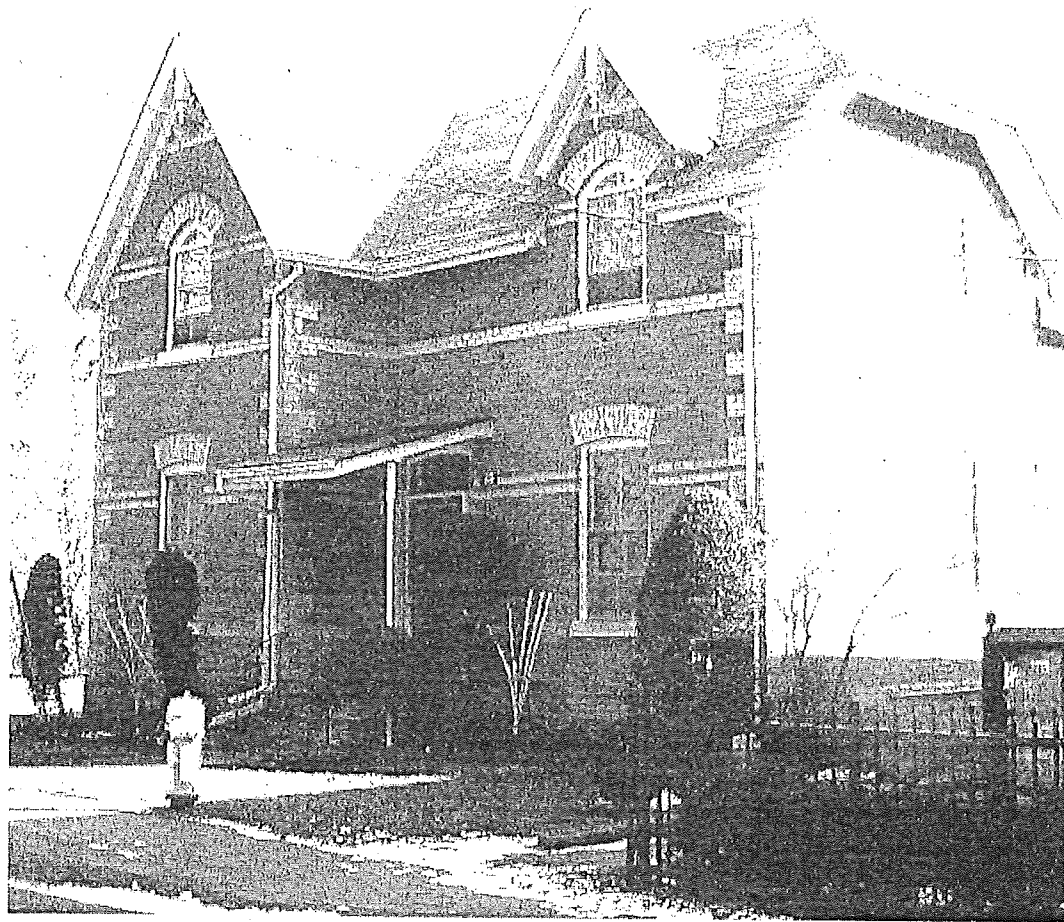
St. Volodymyr's Rectory on Church Lane shows banding (not soldier coursing!), quoining, and voussoirs in contrasting brick.
