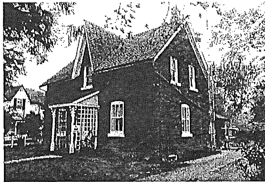
16 John Street: Victorian (porch demolished)
