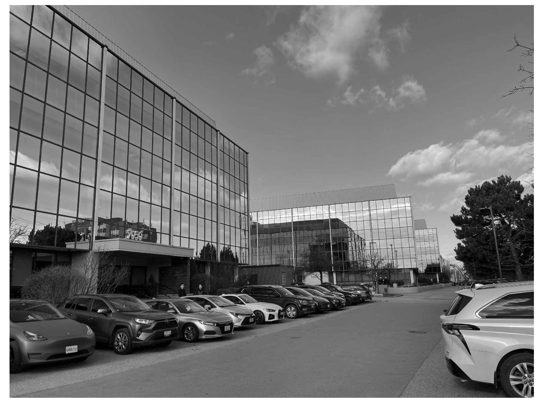
EXISTING OFFICE BUILDING 7050 WOODBINE AVE
