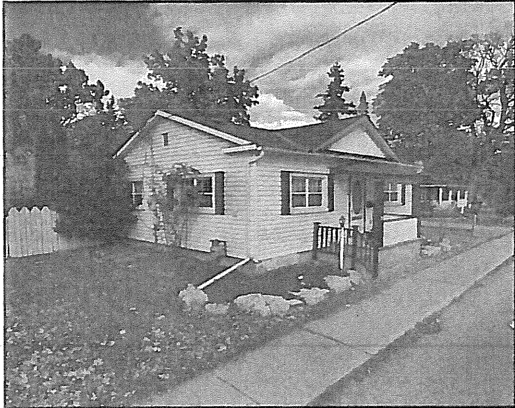
Figure 2- Photograph of the Existing Heritage Dwelling
