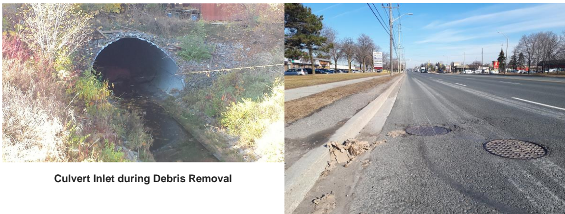
Road Settlement along Culvert Alignment
