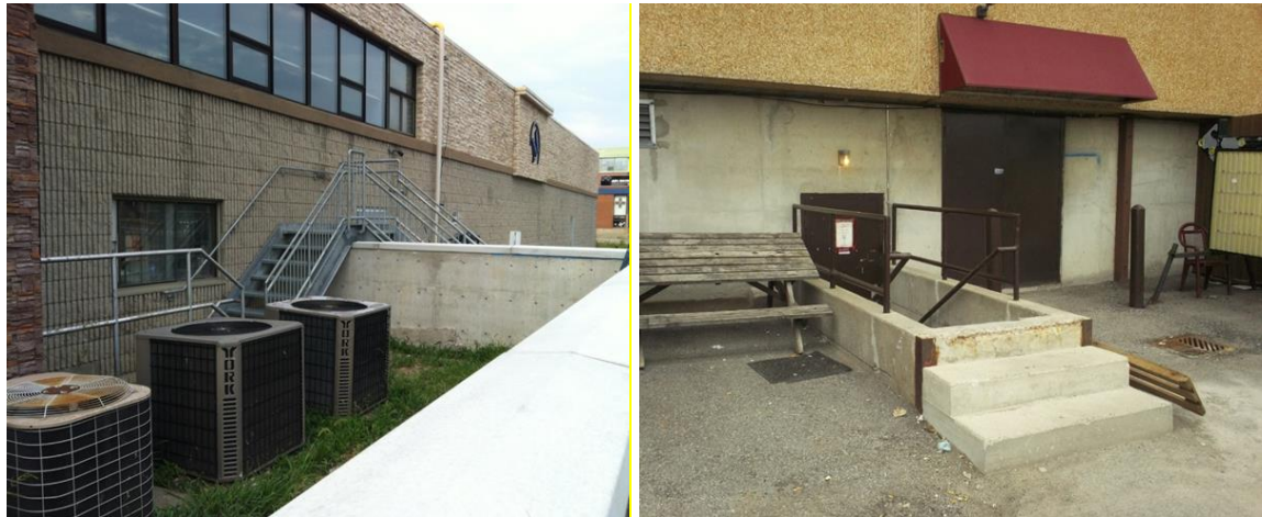
Figure 3-4 Flood Proofing Examples
