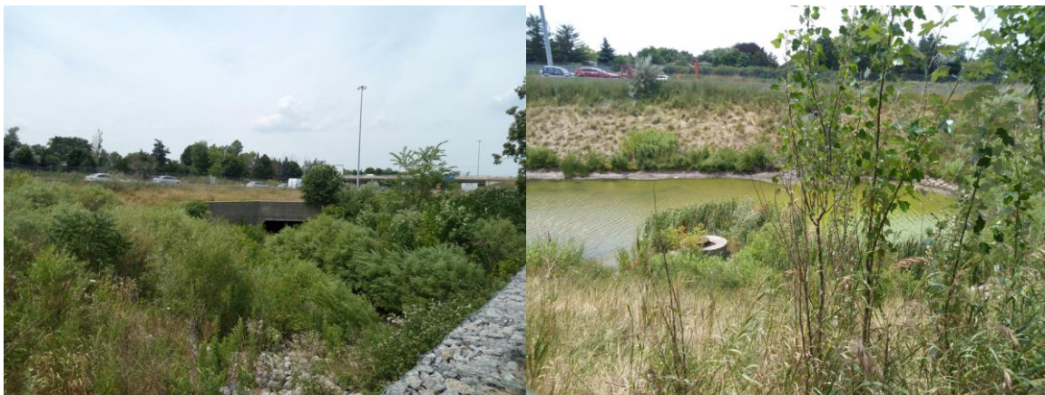
Looking West to Highway 404 Culvert Inlet
