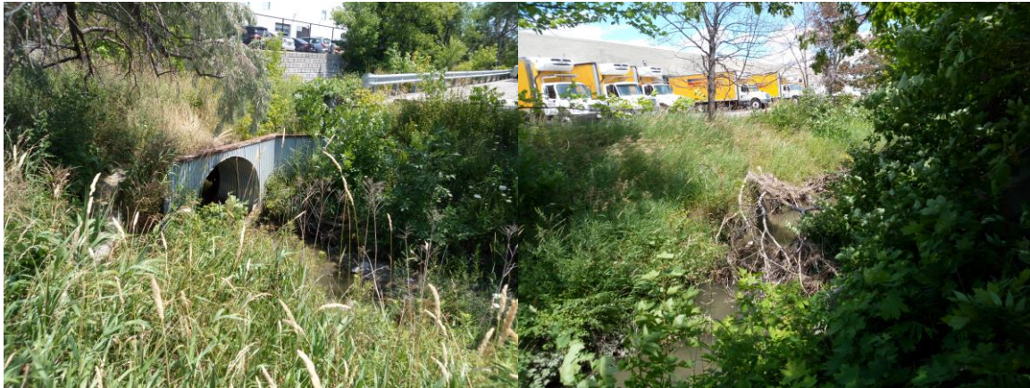
Outlet of Culvert CU10 at 90° Bend
