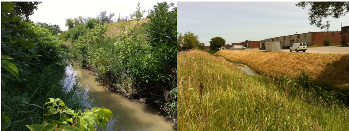
Steep, vegetated side slopes behind 210 Denison Street Recent channel rehabilitation at 130 Denison Street
