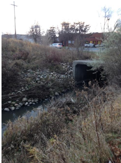
Steelcase Road West Culvert Inlet
