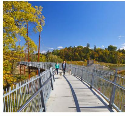
The Milne Creek and Milne Dam Cable-Stayed bridges received a total of 169 votes on Your Voice Markham, winning the People's Choice Award. With a span of 58 metres and 142 metres, respectively, the bridges were designed to minimize disturbance to the natural environment while providing an experience of the valley landscape. They are iconic features of the Markham Rouge Valley Trail that connect neighbourhoods within Markham.
