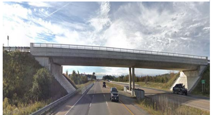
Image 143. Looking south into Markham on Highway 404 at the 19 th Avenue overpass
