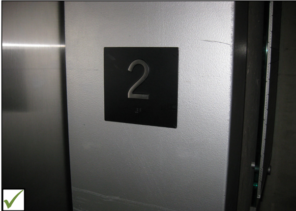
Tactile elevator car identification sign.
