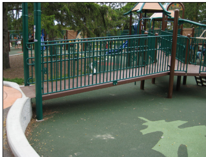
Ramp connected to elevated play components.
