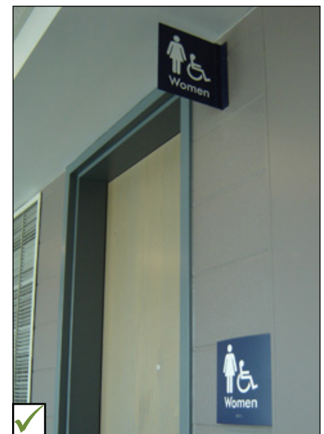
Example of accessible signage to identify accessible washroom.
