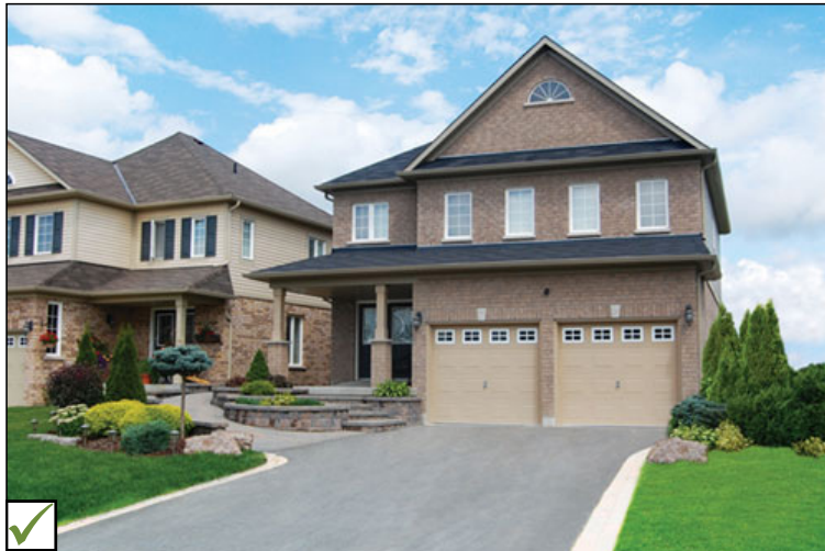
Example of residence with gradually sloped accessible route to main entrance.
