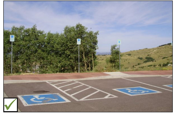
Accessible parking spaces and access aisle.
