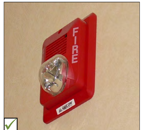
Example of combined visual and audible alarm signals. Public facilities should have both visual and audible fire alarm systems strategically located.
