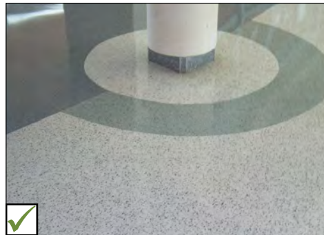
Where structural column / support is within accessible route, colour contrasted floor surface at base is beneficial for all users.
