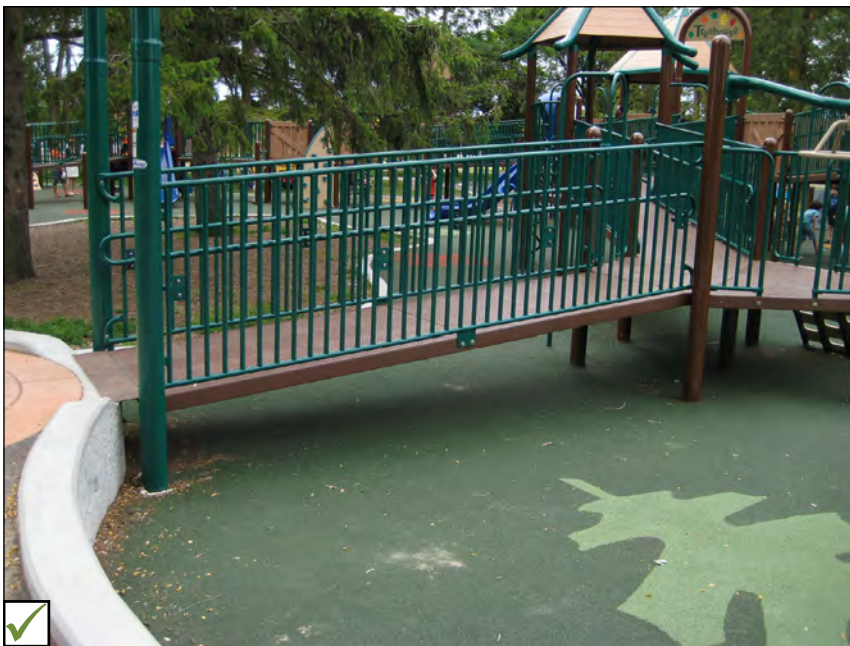
An example of accessible entry / exit point and accessible route leading to elevated play components.
