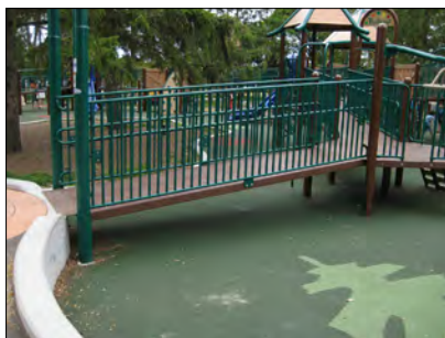
Ramp connected to elevated play components.
