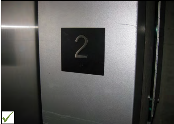
Tactile elevator car identification sign.
