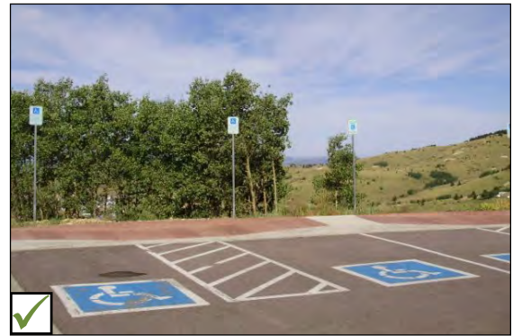
Accessible parking spaces and access aisle.
