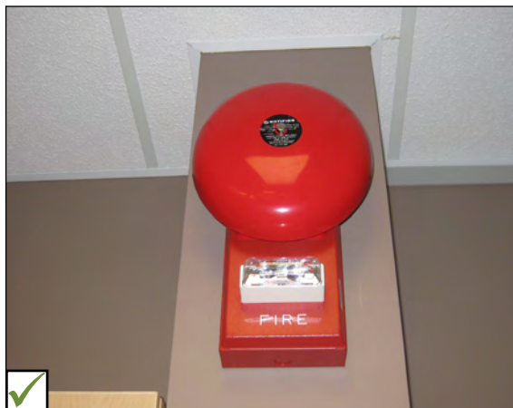
Example of combined visual and audible alarm signals. Public facilities should have both visual and audible fire alarm systems strategically located.
