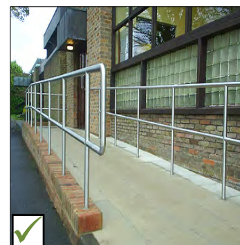
Figure 7c: Handrail Returns to Floor
