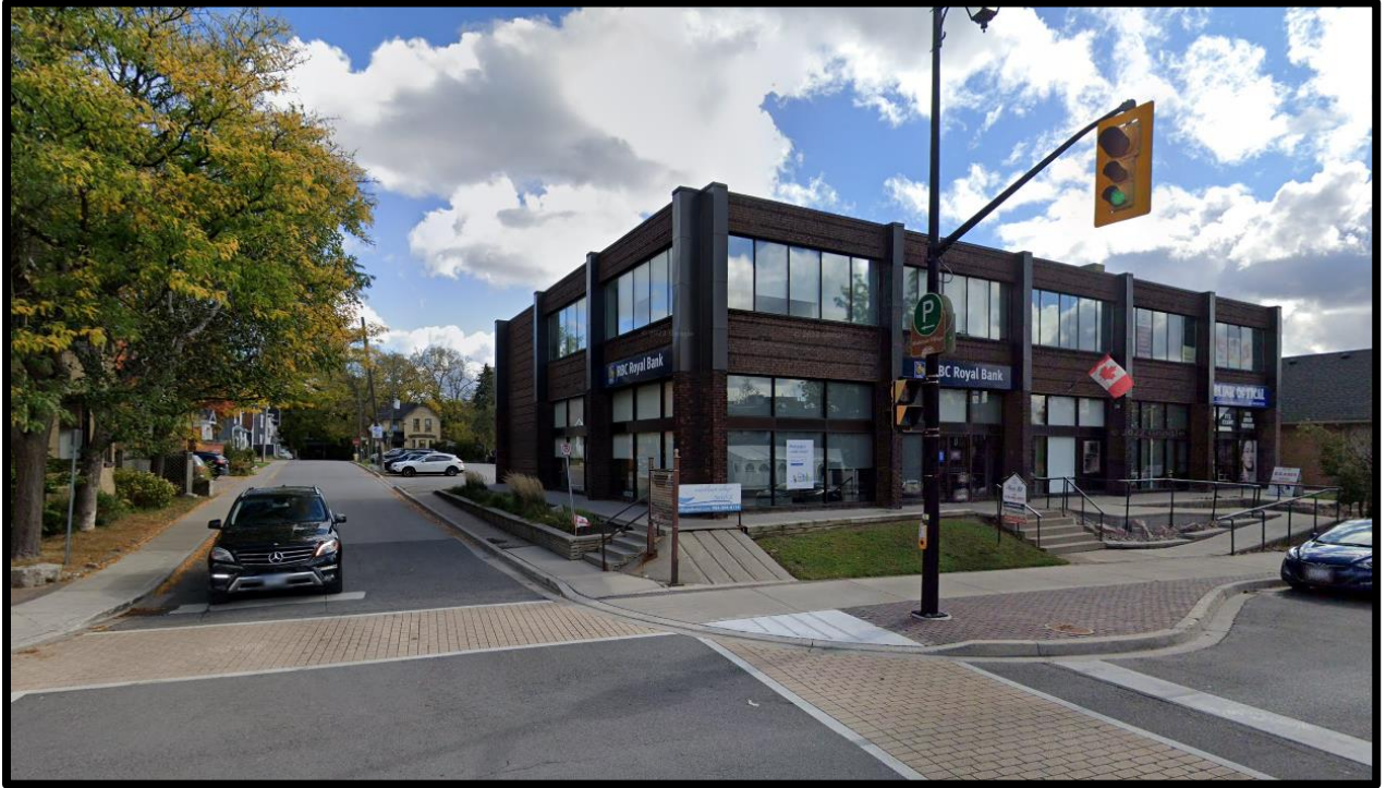
FIGURE 2- PHOTOGRAPH OF THE EXISTING BUILDING
