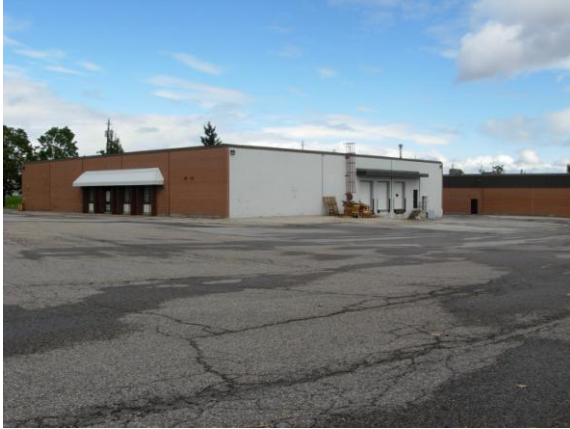
Figure 37: Example of Older ELE Building with Low Ceiling Height
