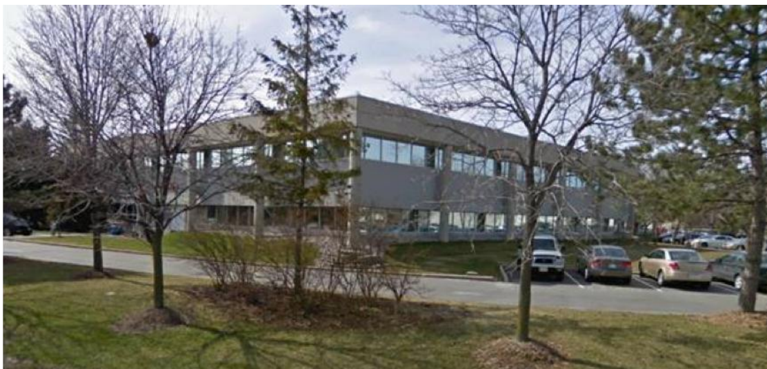
Figure 2: Example of Office
