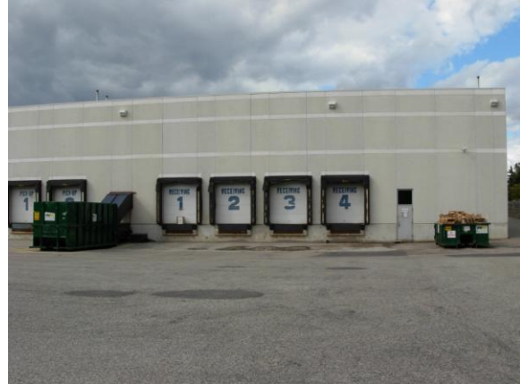
Figure 38: Example of Modern ELE Building with High Ceilings
