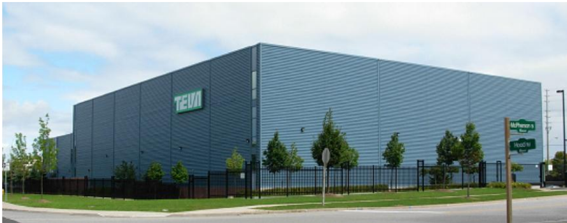
Figure 1: Example of Industrial/Warehouse ELE
