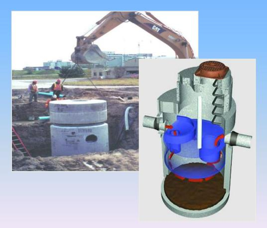
An oil / grit separator is an underground structure connected to the storm sewer to improve stormwater quality by removing contaminants from the stormwater such as grease, oil, mud, sand and trash.
