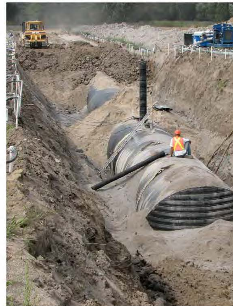
A huge cistern below field areas collects storm water
