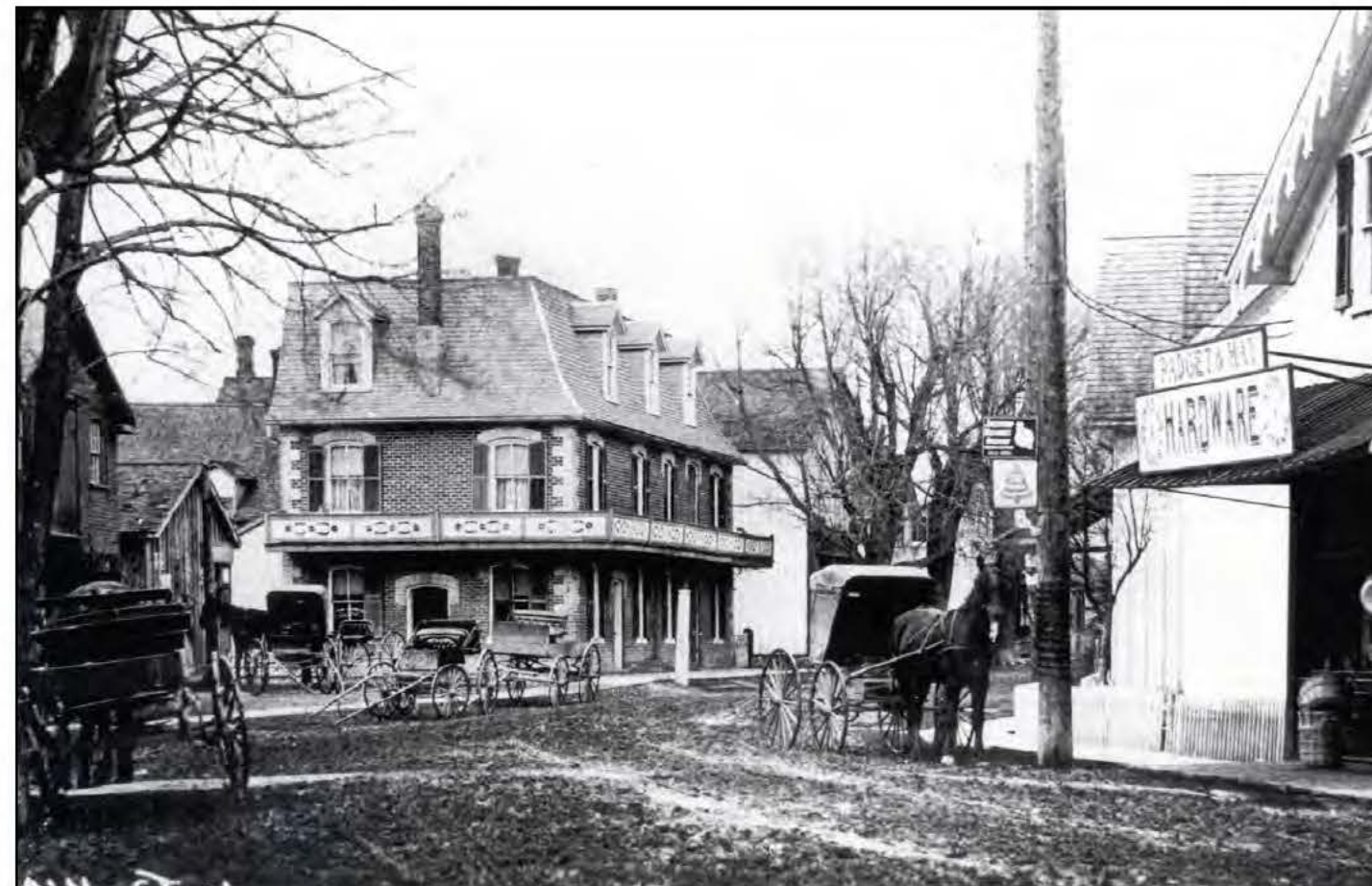
View north on Main Street : The Queen's Hotel, the center of Village life is prominently featured at the bend in the road providing terminating views north and south.
