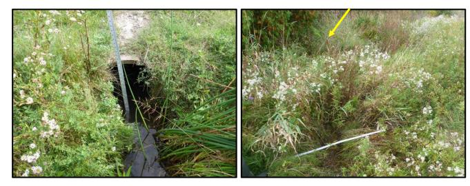
Surface Flow - Photo 61 (Location 59) Existing 500 mm culvert under laneway crossing.
