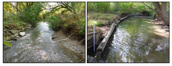
Photo 2 BR-2. Downstream view of general channel conditions. Note stone bank protection on left bank.
