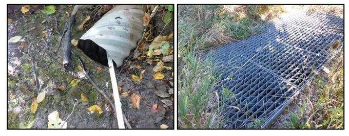
Surface Flow - Photo 67 (Location 65) Existing 300 mm CSP culvert.
