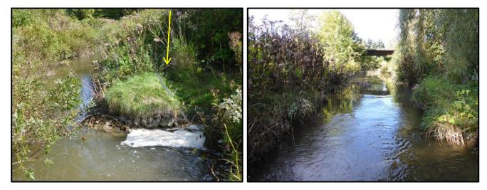
Photo 21 BR-3. Looking downstream at outflanked and undermined gabion basket on right bank.
