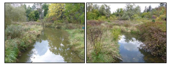
Photo 1 BR-1. Downstream view from pedestrian trail bridge at upstream reach extent. Note widened channel due to backwater from downstream Toogood Pond.
