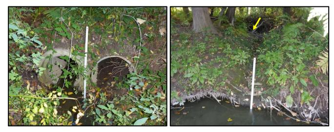
Surface Flow - Photo 81 (Location 79) Upstream view of existing twin culvert under laneway crossing of surface drainage feature.
