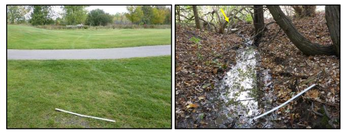
Surface Flow - Photo 63 (Location 61) Downstream view of potential overland conveyance area across the existing fairway. Surface drainage feature is piped.
