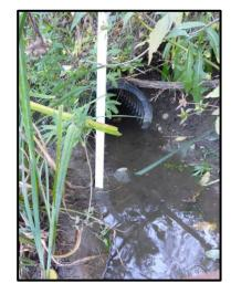
Photo 31 (Location 30) BR-5. Tile drain outlet on right bank.
