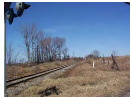
Existing rail corridor in Markham
