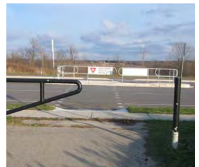
Example of a pedestrian crossing with refuge island, Waterloo, Ontario.
