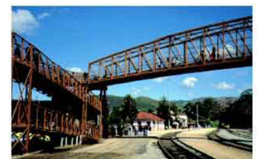
Examples of ramped type bridges
