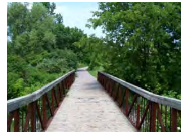
Existing Flat / Linear Pathway and Trail Bridges, Town of Markham
