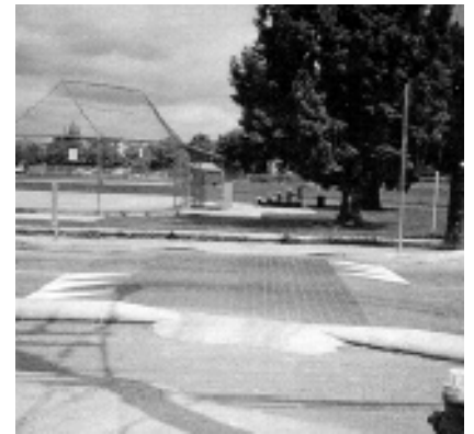
Example of a raised crosswalk. Source: Canadian Guide to Neighbourhood Traffic Calming. TAC (1998)
