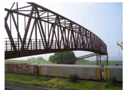
Example of a trail bridge over an active railway line, Port Hope, Ontario, 2006. (Photo: Eagle Bridge)
