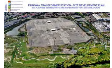
The award winning hydro transformer site on 14 th Avenue provides a diverse pathway experience connecting urban areas to naturalized valleys and open meadows.
