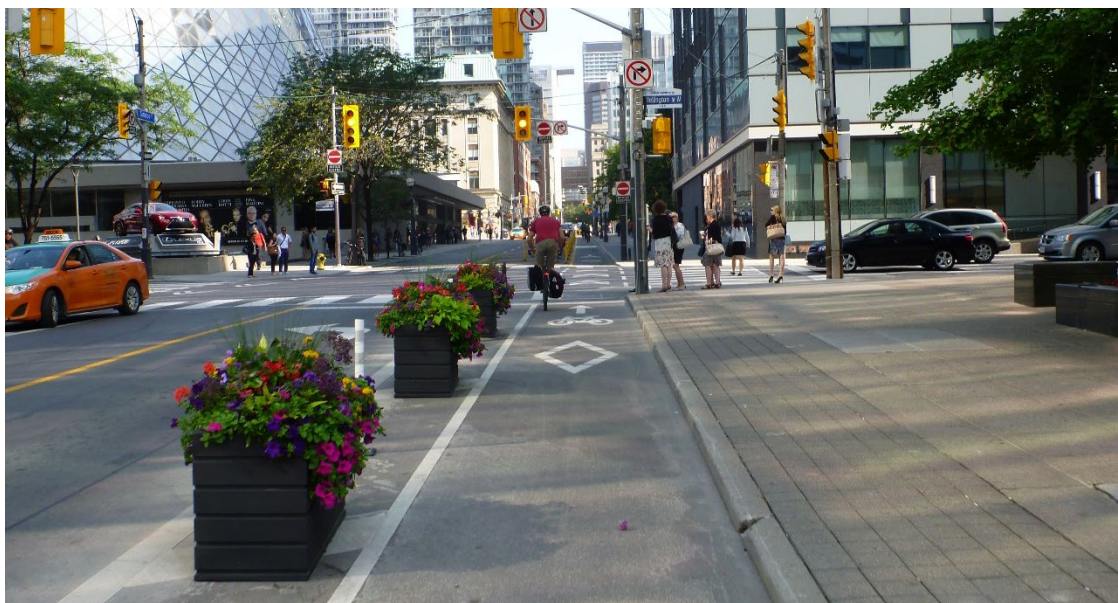
Exhibit 4.1: Example of a Protected Bike Lane
