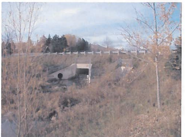
Culvert barrier - Applewood Creek
