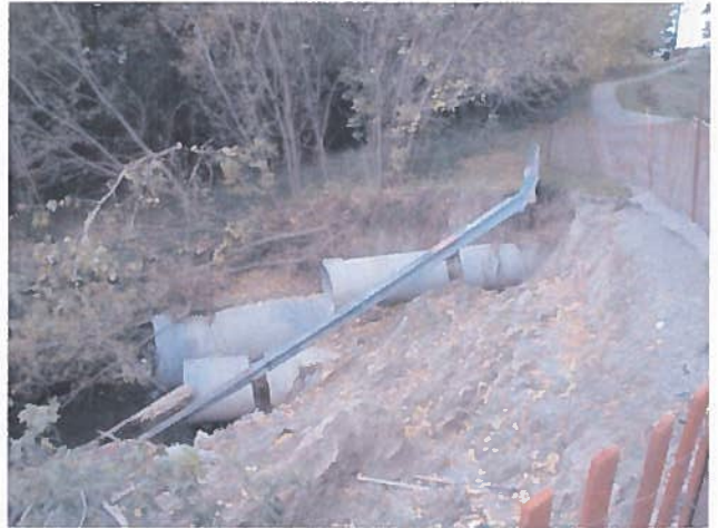
Walkway crossing - Pomona Mills Creek
