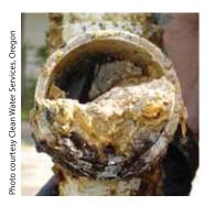
These substances stick to the inner surface of the sewer pipes, harden over time and can cause a sewage backup into your home or on your street.
