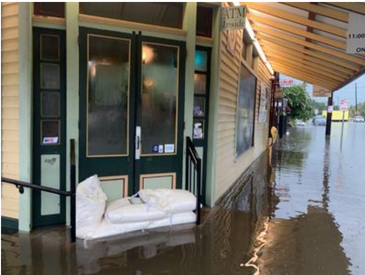
with sandbags (source: nola.com )
