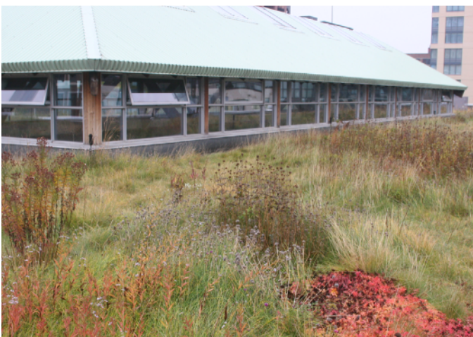
Reflections on green roofs may only reach a few metres above the roof Photo by Brian Roth
