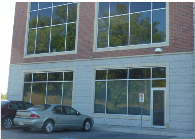
Generally collisions occur from the ground to the top of reflected trees (16m)
