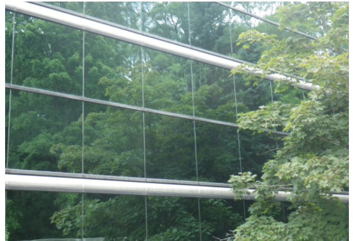
Birds may fly into glass that reflects vegetation Photo by North-South Environmental Inc.
