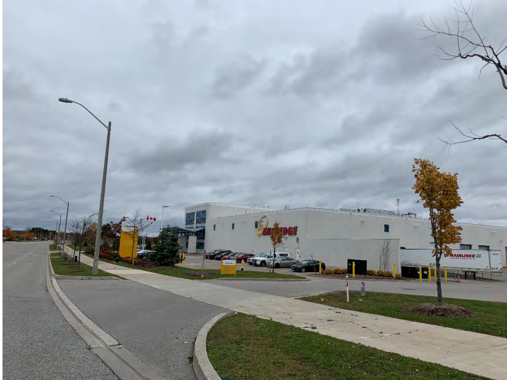
Photo 17: View towards the northeast of the Enbridge facility at 101 Honda Boulevard. Two ASTs were observed at the southeast corner of the property.
