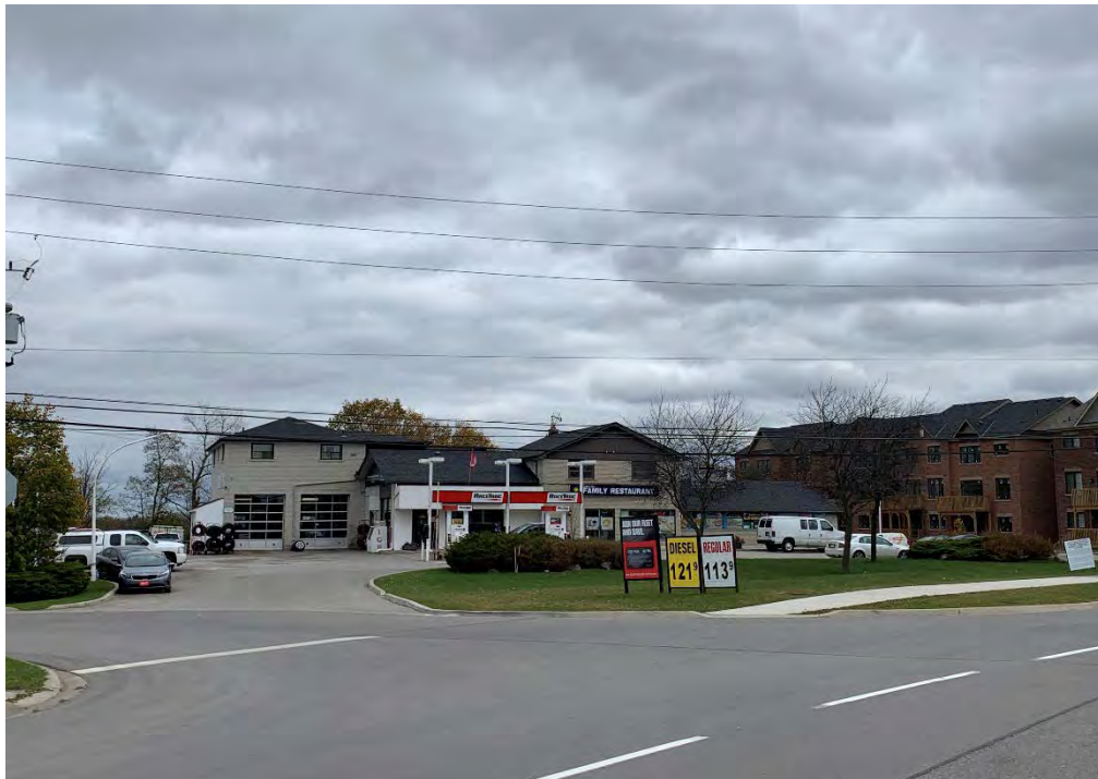
Photo 18: View towards the east of the RaceTrac gas station and Victoria Square Service Centre at 11087 Woodbine Avenue. Covers for USTs were observed near the gas station pumps.
