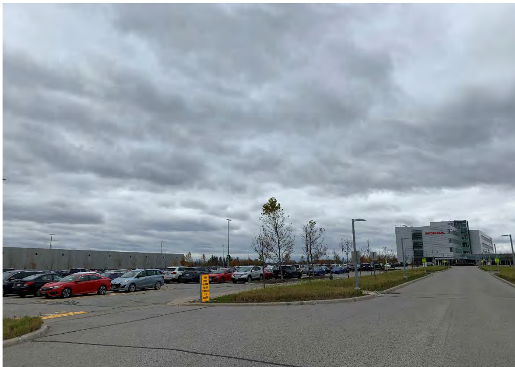
Photo 16: View towards the west of the Honda Canada facility at 180 Honda Boulevard. An office building was observed on the property. A second building was observed which may involve vehicle parts assembly and/or manufacturing.
