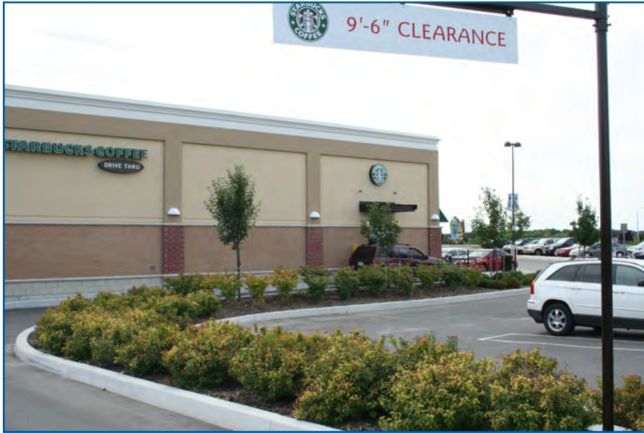
Figure 4.6c: Starbucks at Highway 407 & 9th Line - provides for appropriate curbs and landscaping which separates the stacking lane from the parking areas.
